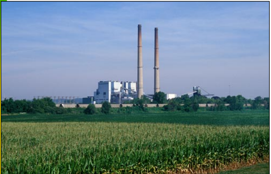
Portage des Sioux power plant near confluence of Missouri and Mississippi Rivers
